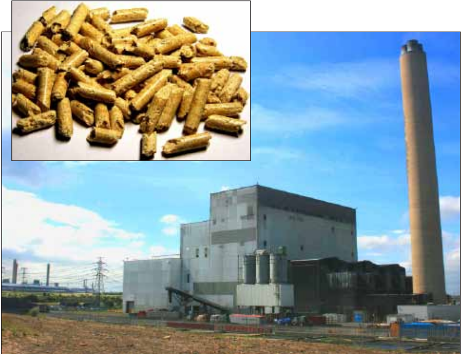
Lynemouth power station, England; formerly coal fueled, then fueled with wood pellets. Credit: Wikimedia, D. Kuru.
